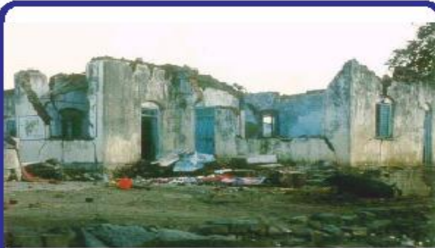
(a) Building with no horizontal lintel band: collapse of roof and walls
