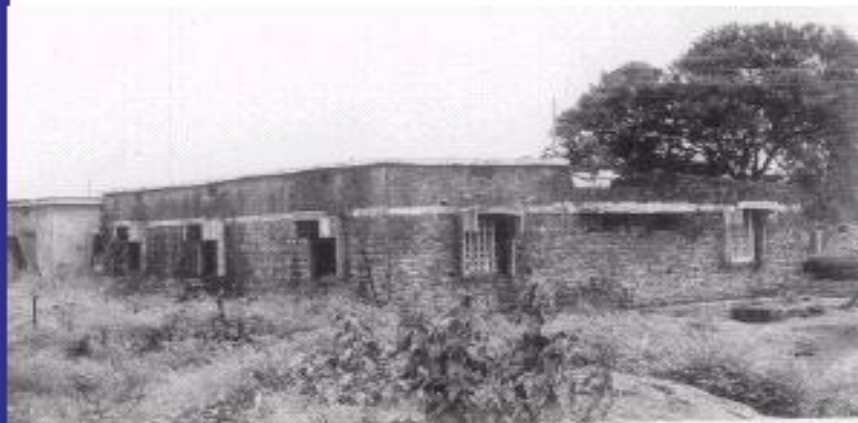
(b) A building with horizontal lintel band in Killari village: no damage
